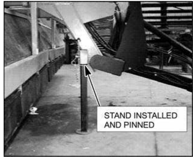
Figure 13. Parking Stand in Lowered Position (Right Side Shown)
