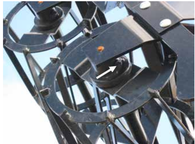
Figure 31. Crumbler Basket Grease Location
